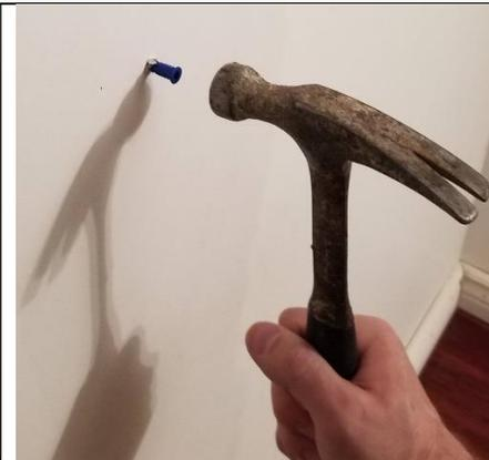
**5** Hammer the anchor into the wall to make it flush
